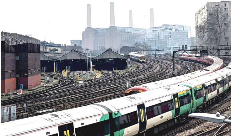
Above is the tangle of lines that enter Victoria station with Battersea power station in the background.
