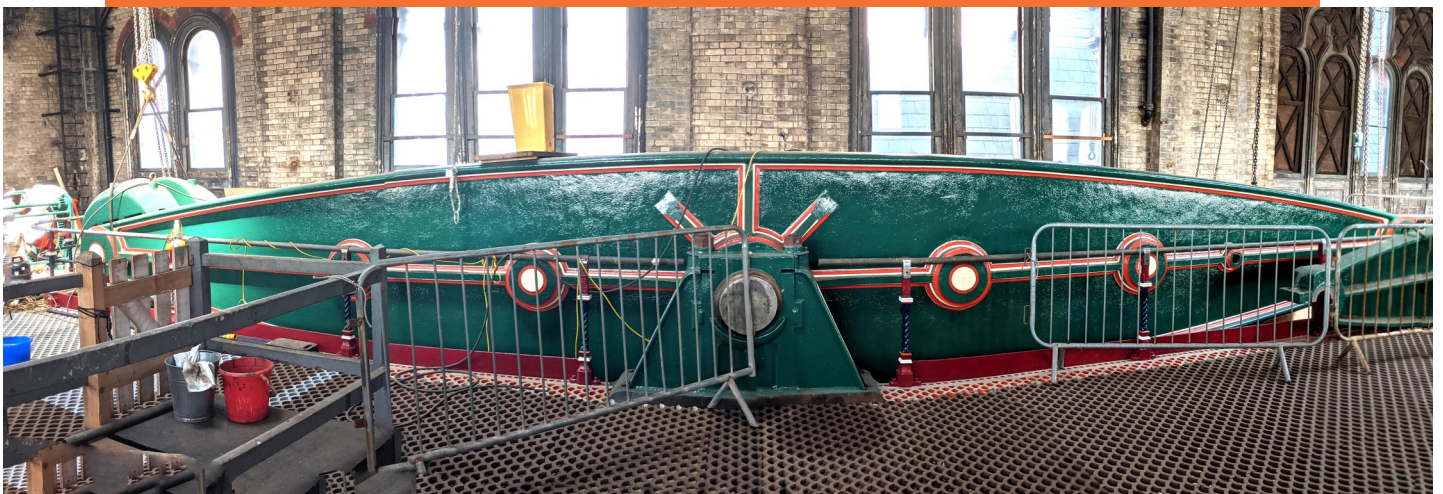
One of the main beams of the Crossness pumping station engines.
